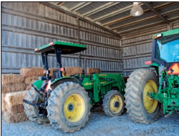
After building the cattle facility, Brewer used guardrails to make a shed.
